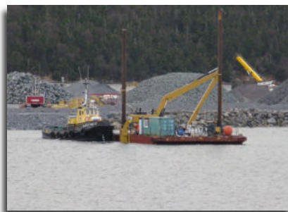
Rock-Reef Under Construction Using Spud Barge
